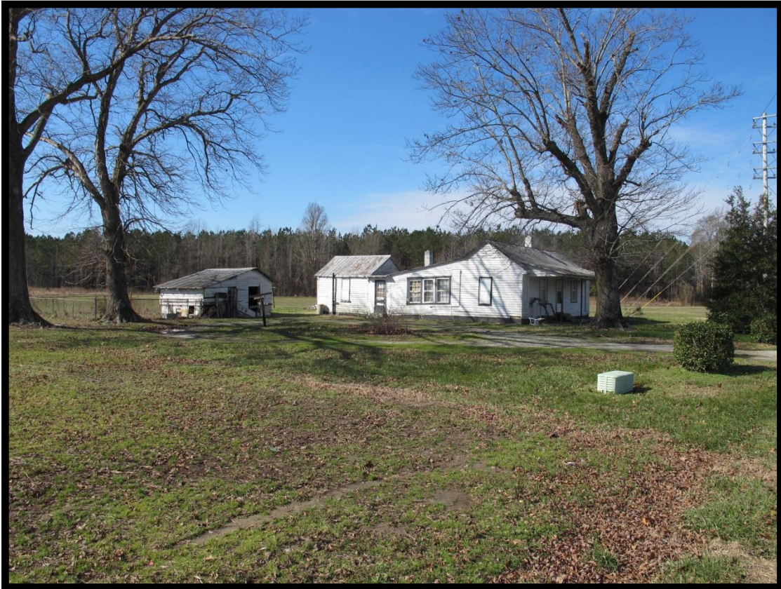
Figure 34: View of House at 4943 Packhouse Road, Looking West.
