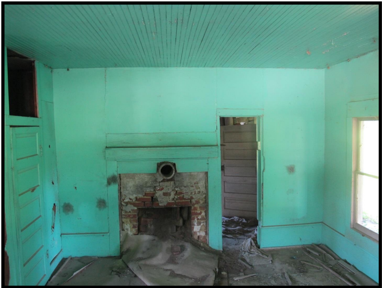
Figure 29: Redmond H. White House (# 012), Interior of East Room Looking West.
