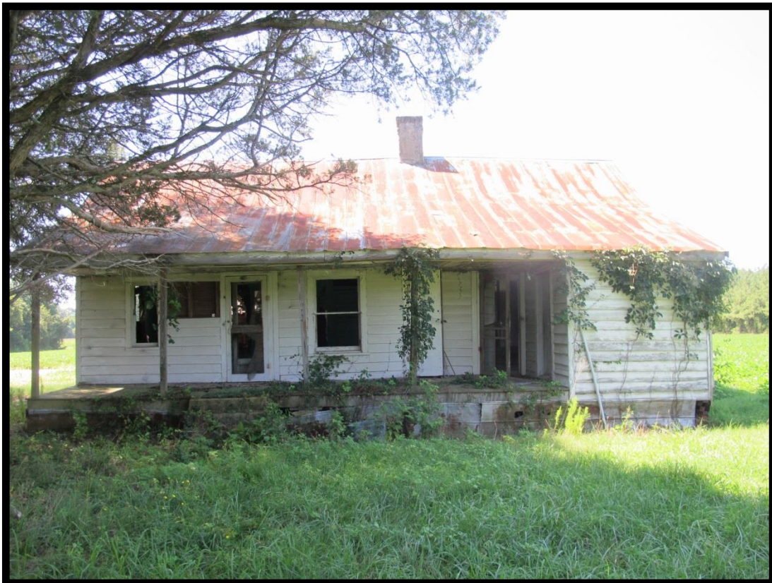
Figure 26: Redmond H. White House (# 012), Looking South.
